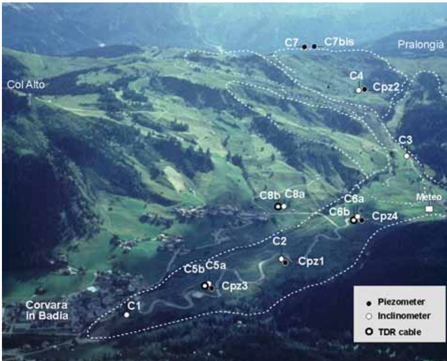
Figure 7. Landslide in Corvara in the Badia valley, indicating the main geotechnical measurement instruments. Example of high intrinsic geomorphodiversity on regional scale
