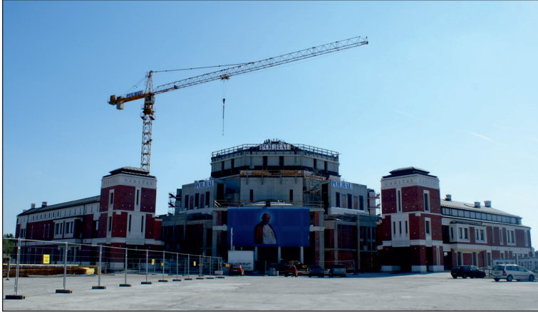
Figure 2. Saint John Paul II sanctuary in Kraków under construction (2014)
