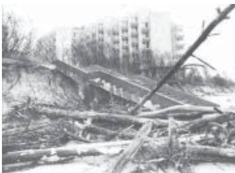
Figure 3. A beach damaged during the storm surge on 3-4 November 1995.
