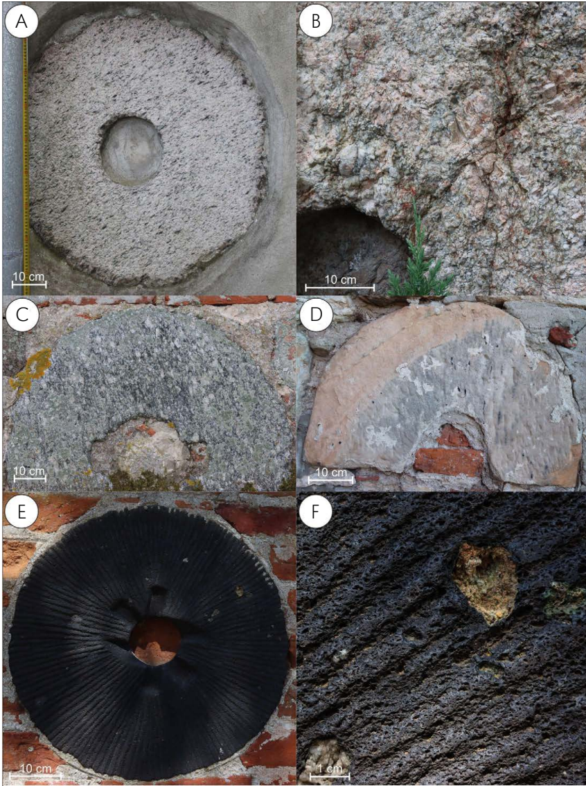
Figure 4. Millstones in church walls; A - millstone or semi-finished product in Bodzanów in Mazovia, leucocratic gneiss (erratic), B - semi-finished product at the entrance to the church in Kraskowo (Masuria), coarse crystalline pegmatite (erratic), C - worn millstone or semi-finished product in Rogiedle (Warmia), gneiss with small crystals (erratic), D - semi-finished product used as building material in the monastery church in Sulejów, sandstone from the vicinity of Wąchock (northern Mesozoic margin of the Holy Cross Mountains), E, F - worn millstone in the ruins of the church in Wocław in Żuławy, porous volcanic rock, most likely imported from the Eifel massif (?). (Photos by P. Czubla)
