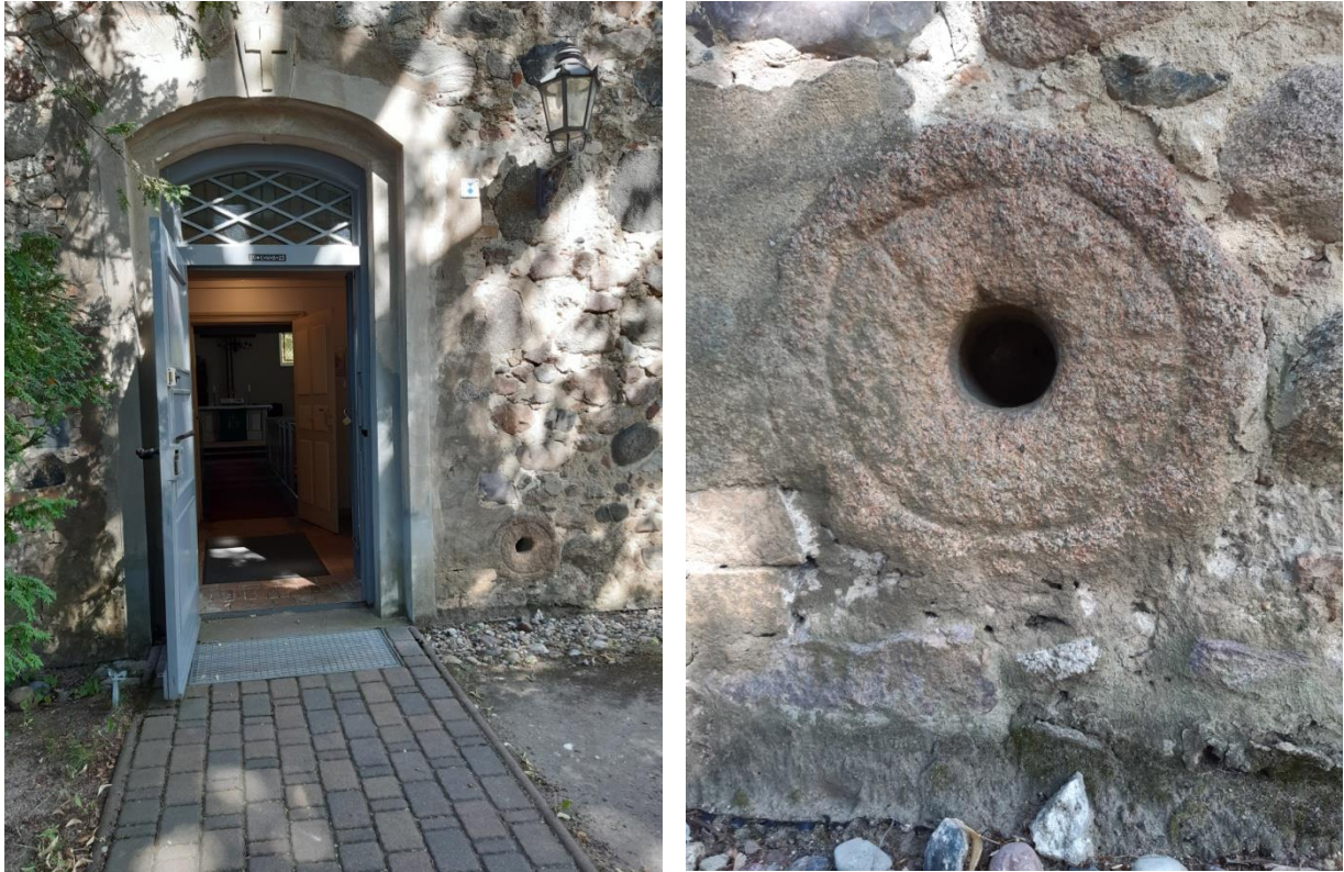
Fig. 13. Millstone embedded next to the portal of the church in Miersdorf (photo by Dariusz Brykała)
