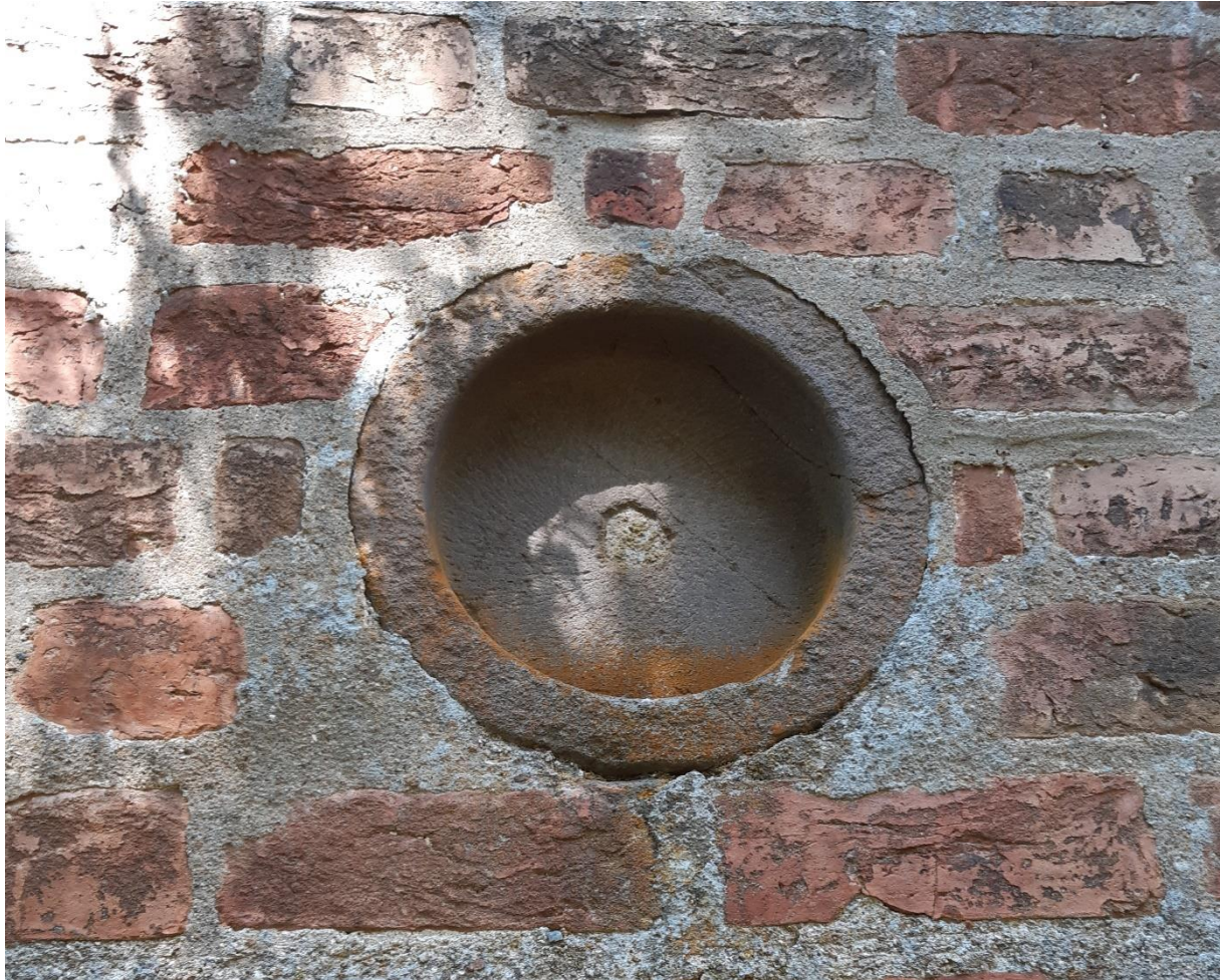
Fig. 1. Hakenberg (Brandenburg), village church. Medieval pot quern of basalt-like lava (diameter 39 cm), secondarily used as baptismal font and since 1875 bricked in the tower (photo by Dariusz Brykała)
