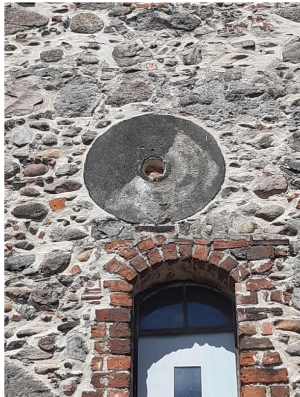
Fig. 10. Millstone embedded in the tower of the church in Rottstock (photo by Dariusz Brykała)
