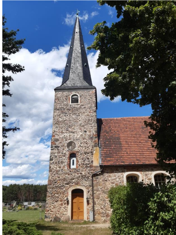
Fig. 9. Tower of the church in Rottstock: view from the south (photo by Dariusz Brykała)
