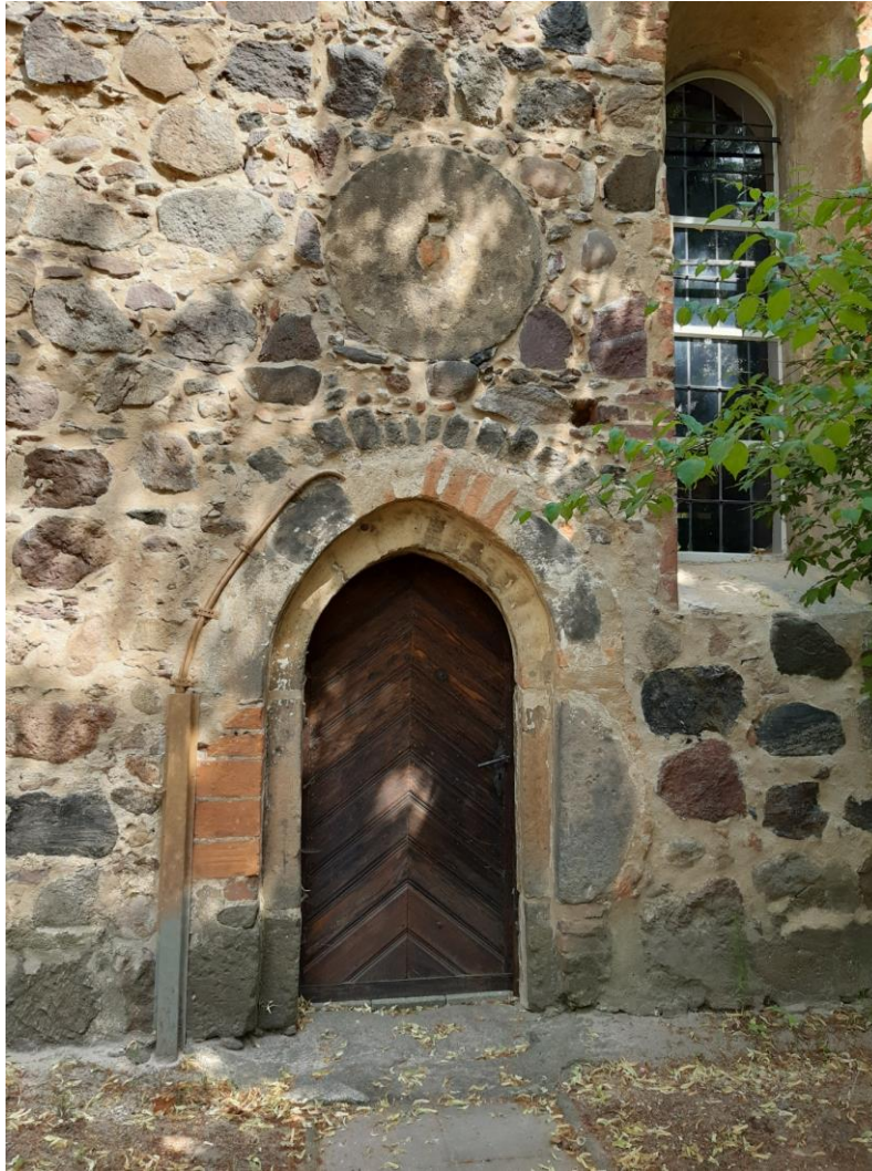
Fig. 7. Location of a millstone and a fragment of a putative half of another millstone embedded in a wall of the church in Gießmannsdorf (photo by Dariusz Brykała)
