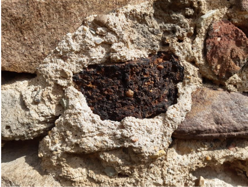
Fig. 2. Piece of bog iron ore in the mortar of the church in Falkenhain (photo by Dariusz Brykała)
