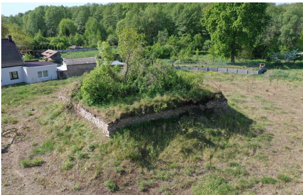
Fig. 8. Relics of the stone tower after the demolition of the site. East view taken in 2022. Photo: H. Augustyniak.
